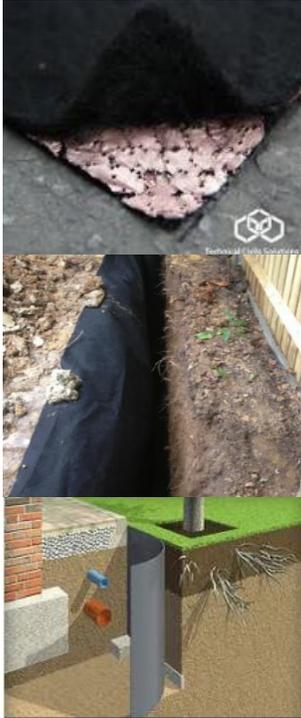
This solution is multipurpose and ideally suited to the current application. Traditional impervious barriers divert rather than stop roots and may block moisture movement. Also, roots getting under such barriers can grow back to the surface. Therefore, the use of this permeable barrier stops roots either by engaging and constricting them or by chemically inhibiting them.
